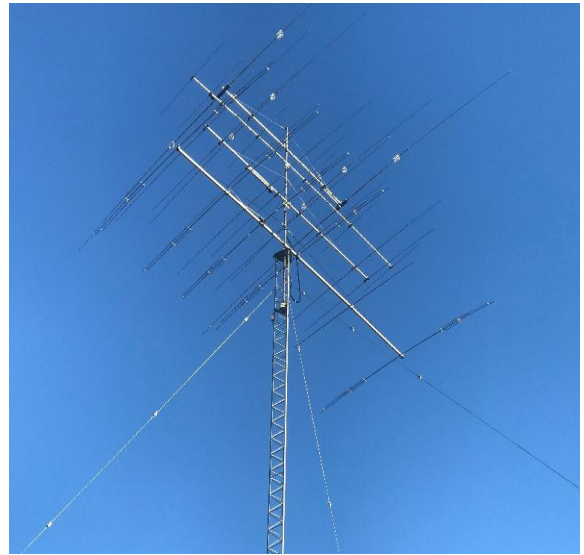
N6AR's antenna system - a 7-element JK six-meter Yagi at 80 feet in the station's "Christmas tree" stack.
