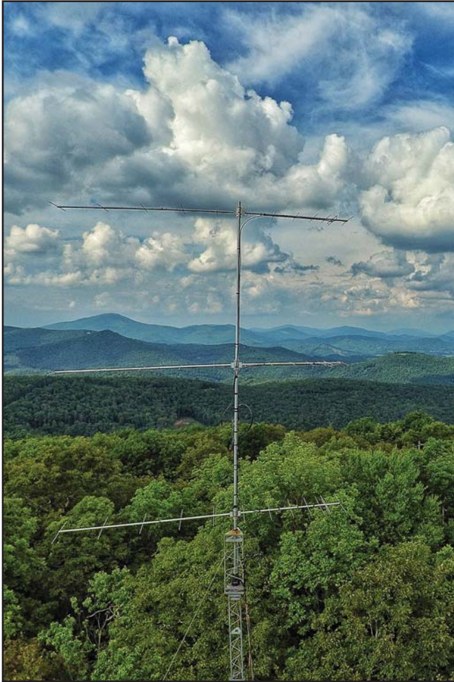
Paul, AA4ZZ, sent in these photos, shot by a drone, of the 2-meter Yagi used for the W4VHF contest station. (Photo by W4GRW)
